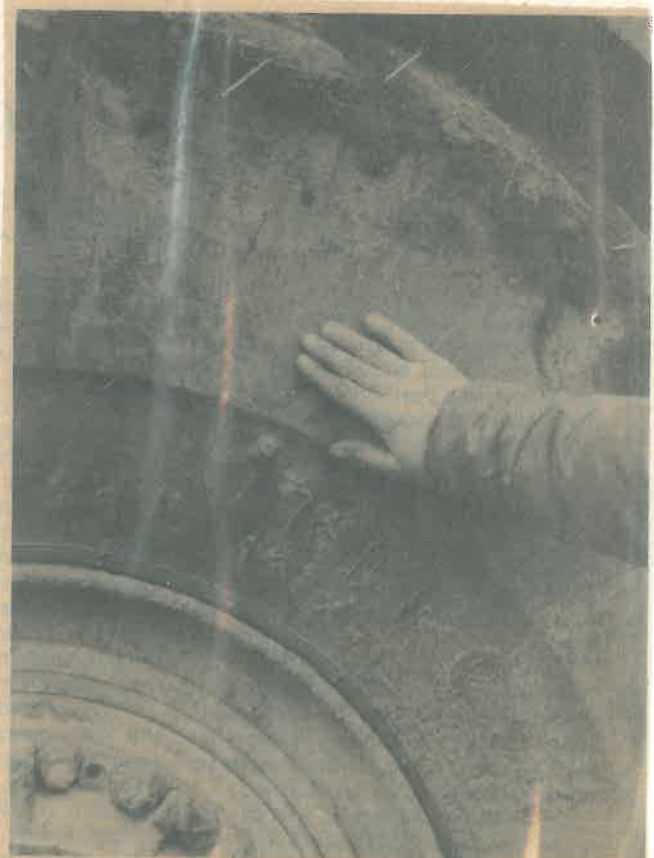
TEMPORARY REPAIRS — Temporary repairs were made on this large tire, and 43 others, after they were punctured in a vandalism incident at the new Borden Bridge construction site early Sunday. The $150,000 worth of tires will have to be replaced but the air leaks were stopped for now by bolts like the one to the left of the hand in the photo.
